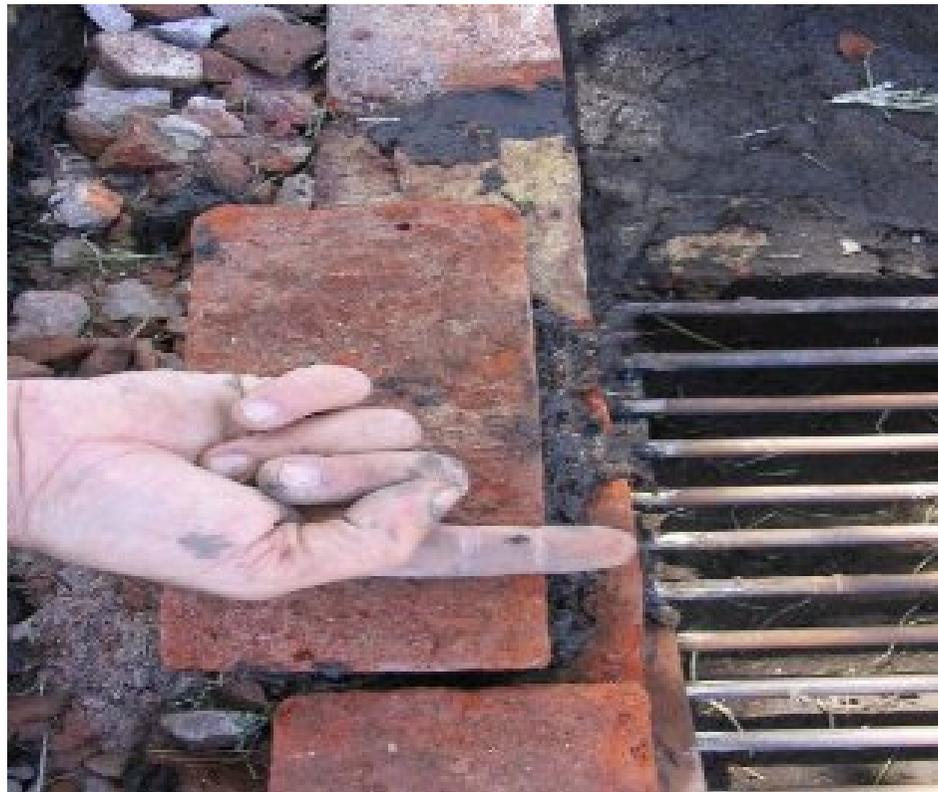
**LA PARED INTERNA SE PUEDE HACER CON LADRILLOS REFRACTARIOS O CON VIDRIO PICADO MEZCLÁNDOLO CON EL BARRO.-**
